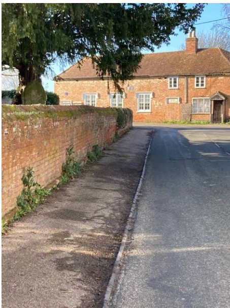
62. To show proximity of ancient wall, blind bend and over-hanging tree. This is corner for War memorial, children's playground and village hall
