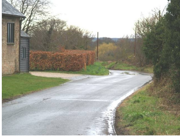
17. This is facing back down Kelvedon Road near the junction with New Road and shows the narrow blind bend.
