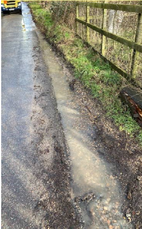
54. To illustrate extensive damage already made as traffic is forced to make passing places
